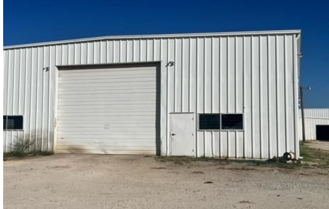
Building 1 - Rear View
